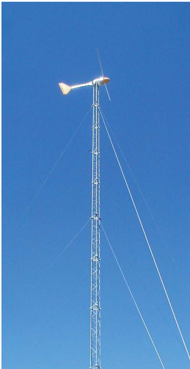
Fixed, guyed towers share characteristics of both tilt-ups and freestanding towers.
