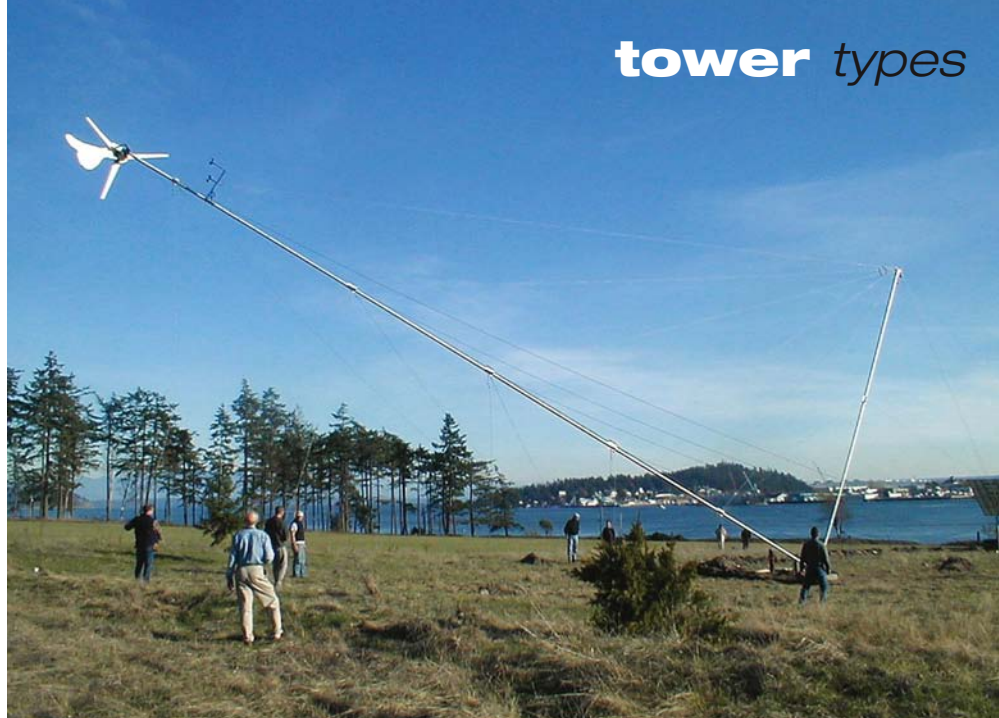
As the gin pole goes down, the tower goes up—tilt-up towers need wide open and level spaces, but make installation and maintenance easy.
