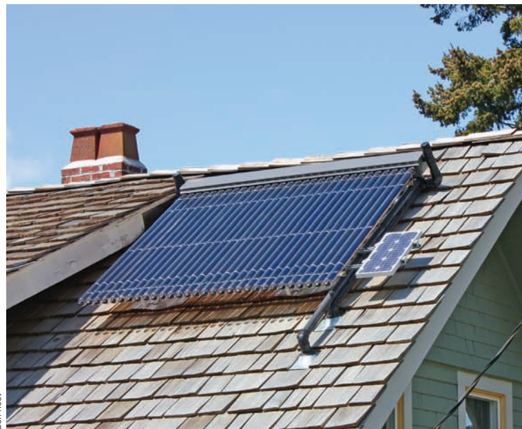
While evacuated-tube collectors are less affected by angle and orientation, mounting them parallel to a steeply pitched roof will improve their wintertime production.
