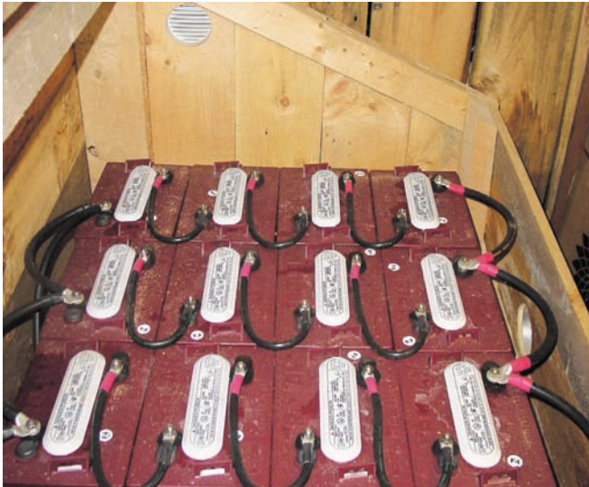
Contained in this simple battery box, three parallel strings of four 225 Ah Trojan T-105 batteries make a 24 V, 675 Ah battery bank.
