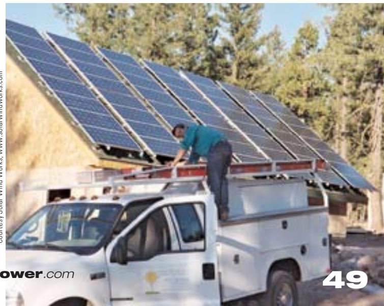
Neal Mock from Solar Wind Works wraps up another system installation.
